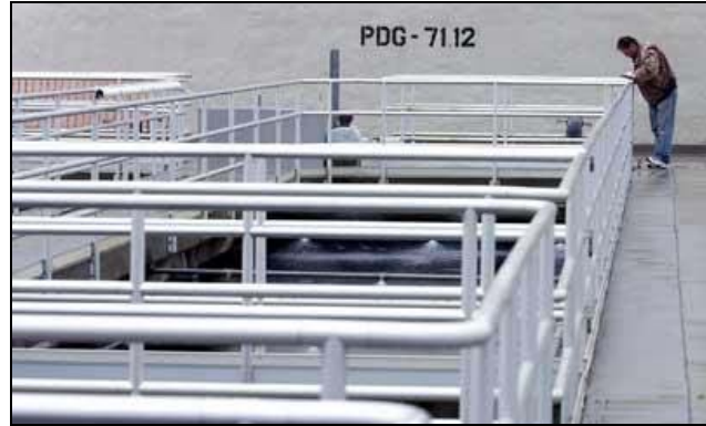
A worker at the Easterly Wastewater Treatment Plant looks over some of the tanks used at the treatment facility.
